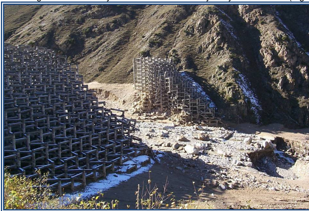
Fig. 9. The dam on the Gerkhozhan-Su river, destroyed by a debris flow in 1999 (photo by I.B. Seinova).
