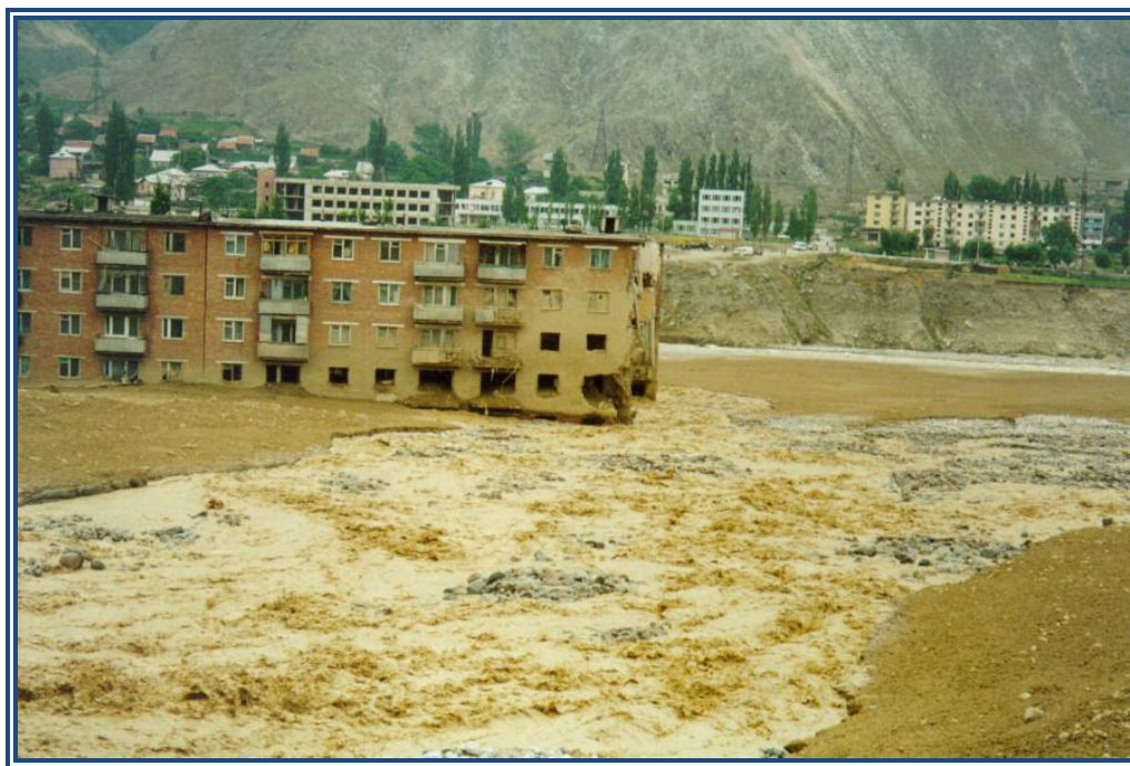
Fig. 10. Residential building in the town of Tyrnyauz, affected by a debris flow in 2000 (photo by S.S. Chernomorets)
