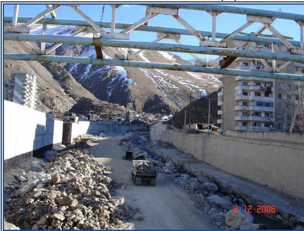
Fig. 11. Reconstruction works on the debris flow control chute in the mouth of the Gerkhozhan-Su river (photo by S.S. Chernomorets)
