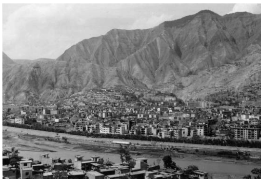
Fig. 2. More than 10 debris flows endangered Wudu city in southern Gansu, which suffered dozen debris flow hazards since the year of 1368
