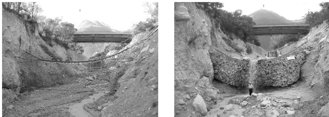
Fig. 2. Flexible ring-net barrier system at the Illgraben before and after filling.
