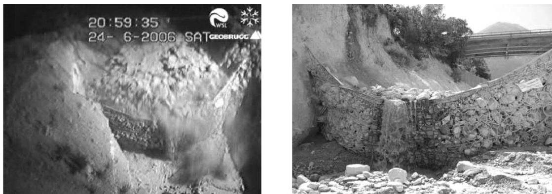
Fig. 3. ROCCO ring-net barrier during and after the 24 June debris flow.
